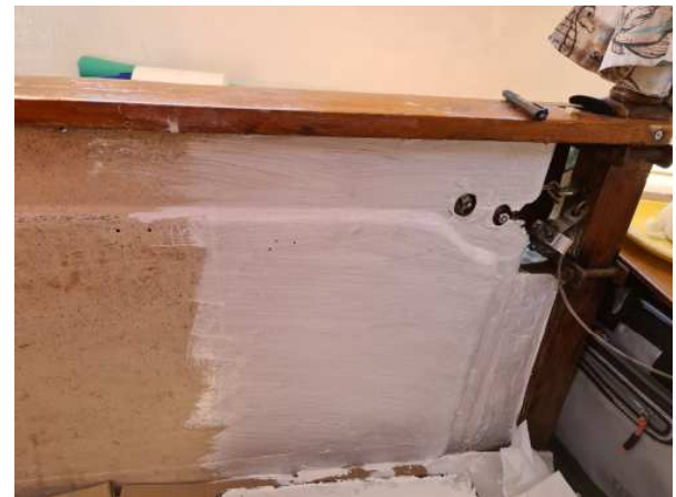
Figure 2 – 1st coat applied over GelCoat
