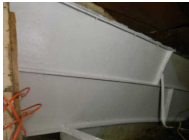
Figure 6 – FloCote over rusty steel treated Feronite Rusty Metal Primer
